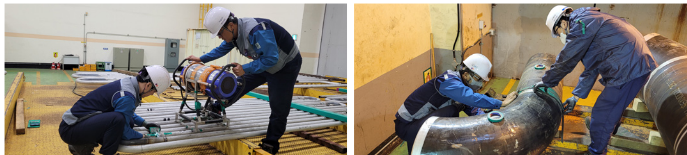
(Example of inspecting the quality of boiler tube welds for power generation, Doosan Enerbility)
